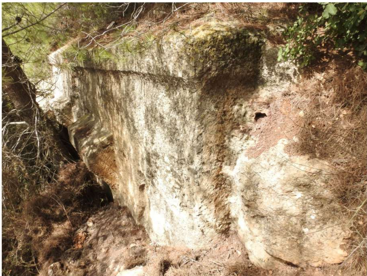
Figure 15. Complex 3: A. Elevation. B. F7, view from the south-west. Elevation by: M. Kahn, processed by: Y. Shmidov. Photo by: H. Shkolnik.
